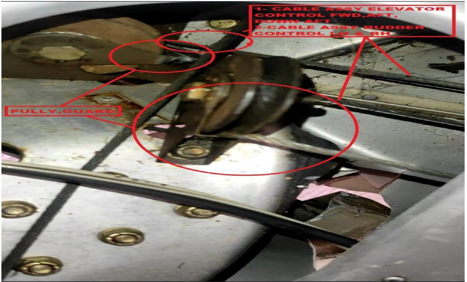
13- Some Pulley, Guard found damaged.
